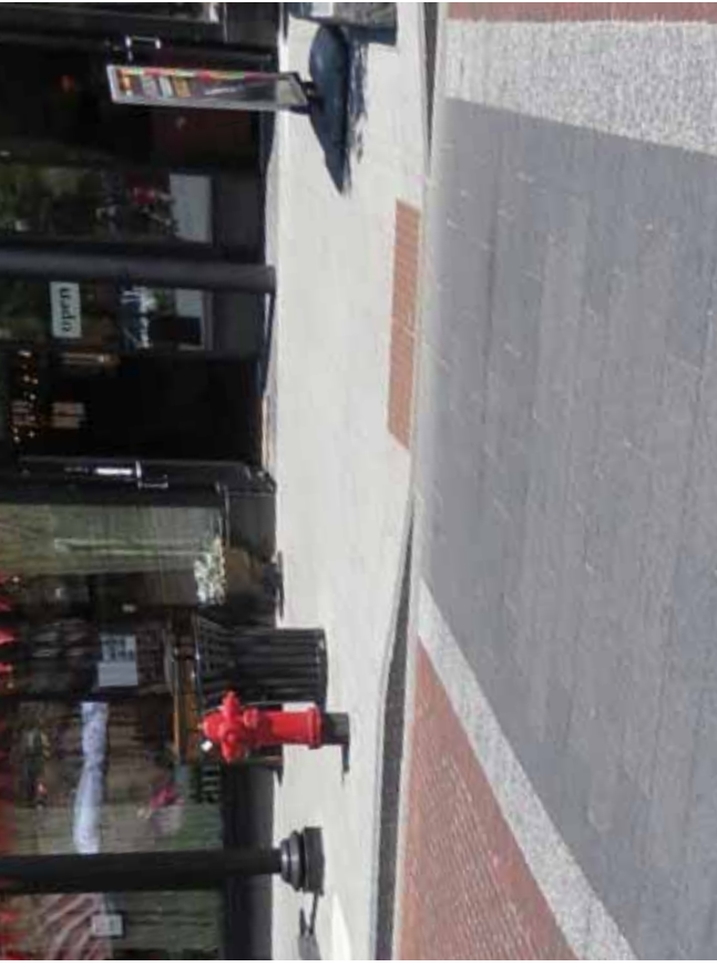
Stone Crosswalk: Thermal cut granite, Oxford Black and Rockville White
