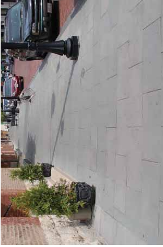
Bluestone Sidewalk: Thermal cut bluestone
