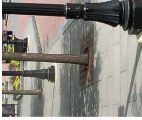
Tree Grate: Garland design by East Jordan, 4'x6' - final size to be determined
