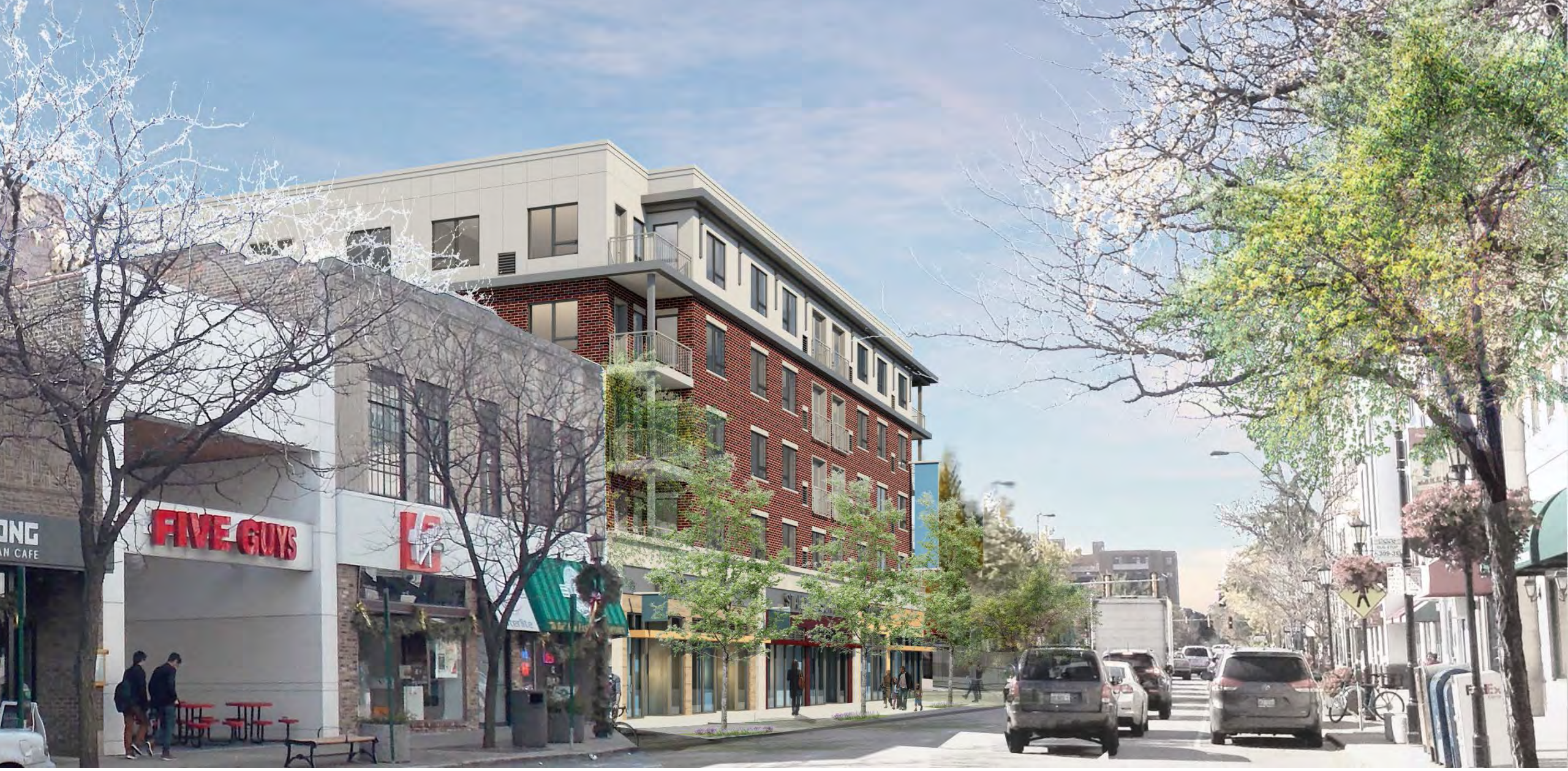
(11) North Building Cornice View Looking West (before)
