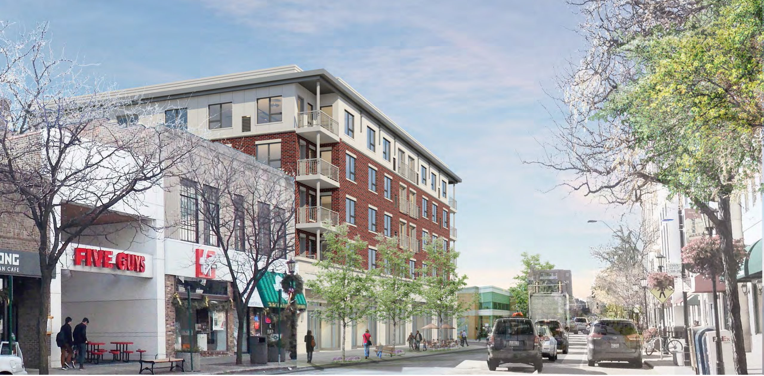
(11) North Building Cornice View Looking West (before)
