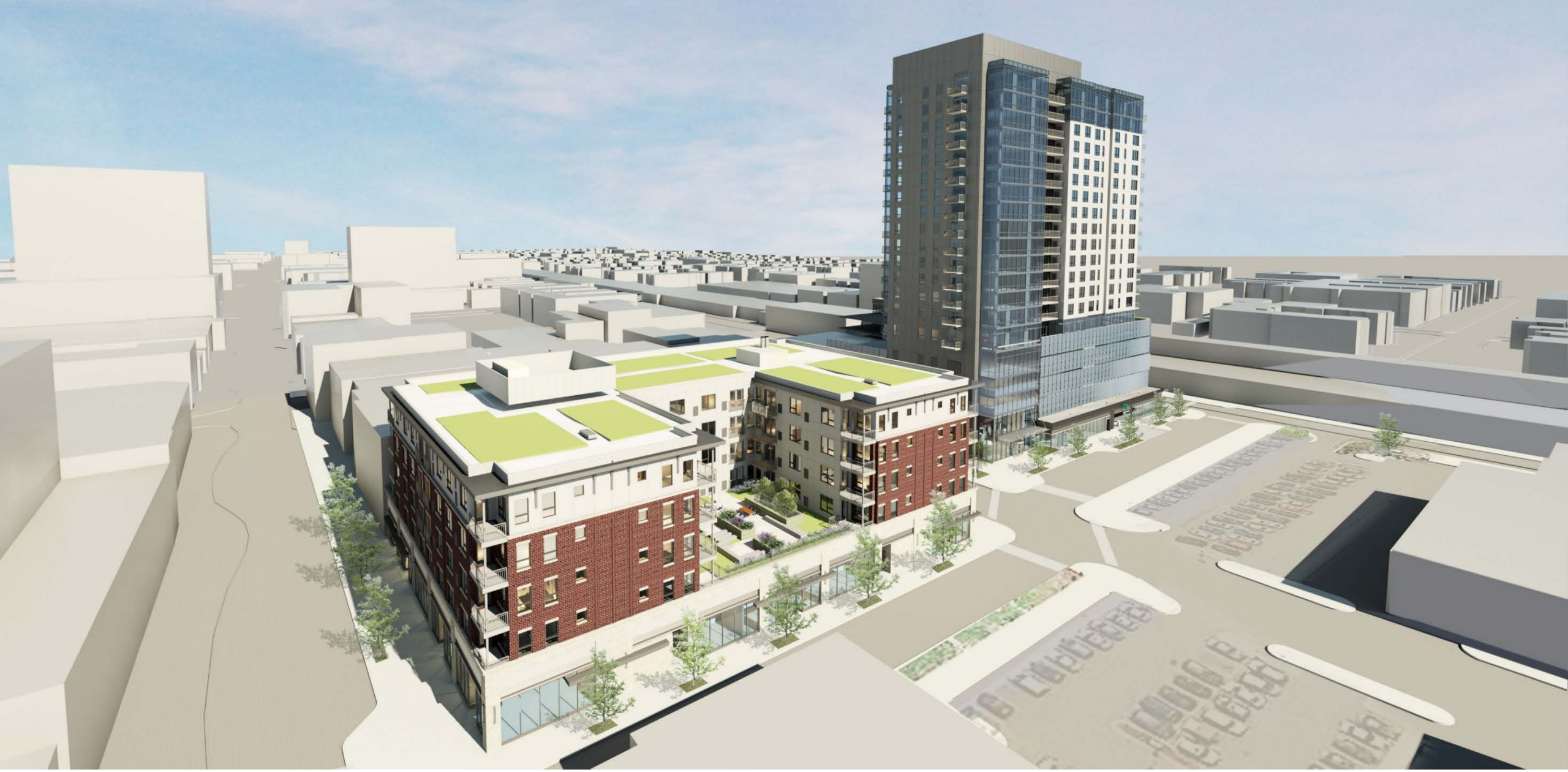
(11) South Building Garage Screen Looking Southeast (current scheme)
