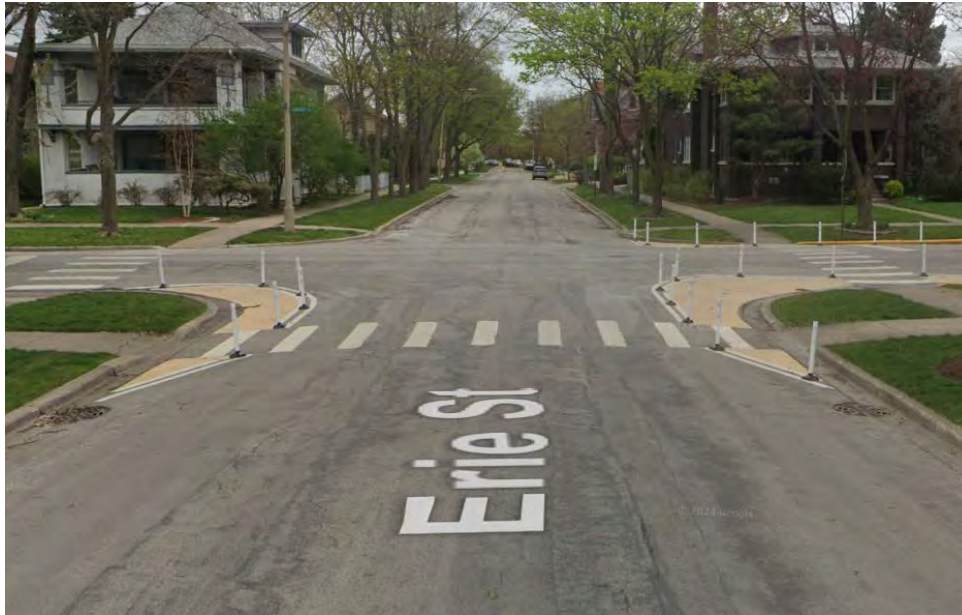
Figure 4. Paint and Post Curb Extension Example
